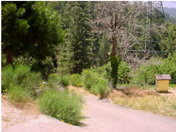
Spanish broom along East Incline Distribution Line at the road to Big Creek Powerhouse No. 1.
