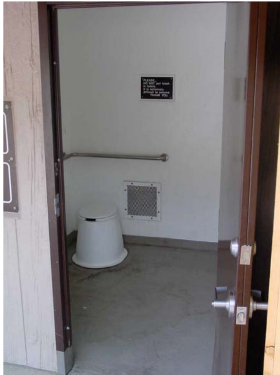
Boat Ramp – Huntington Lake (USDA-FS), Parking Area Restroom Stall – ADA Compliant
