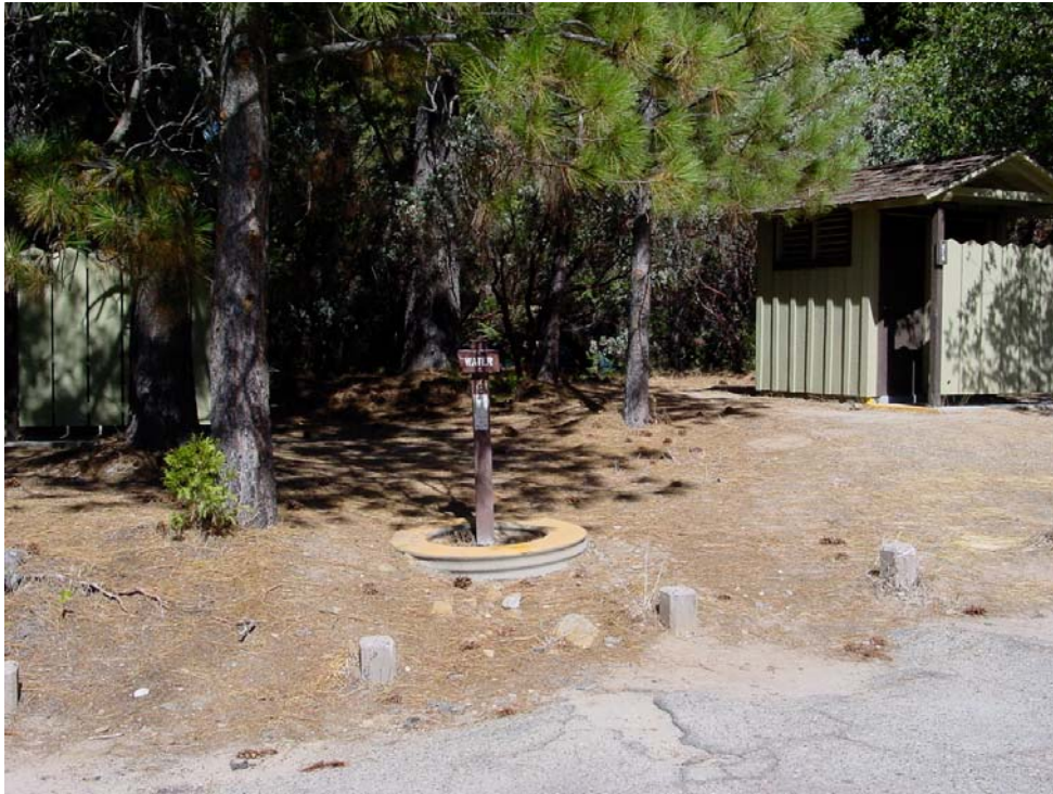
Mammoth Pool Campground, Water Spigot and Restroom – Non-ADA Compliant Features
