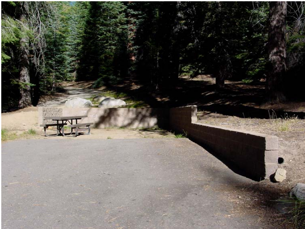
Catavee/Kinnikinnick Campgrounds, Campsite Created with Retaining Walls – ADA Compliant
