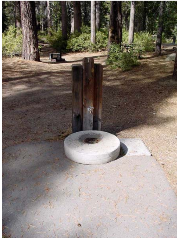
Deer Creek Campground, Water Spigot – ADA Compliant Design
