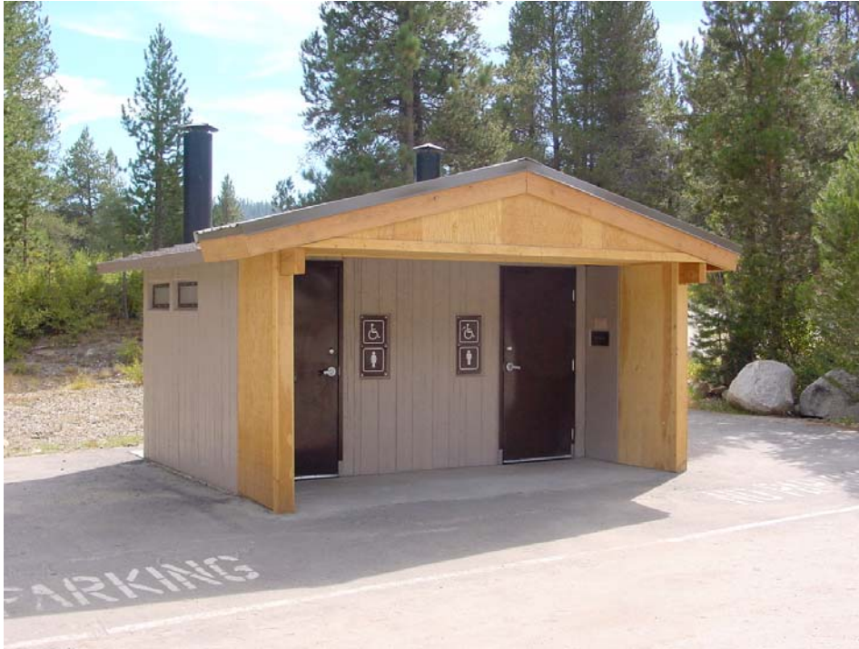
Boat Ramp – Huntington Lake (USDA-FS), Parking Area Restroom – ADA Compliant
