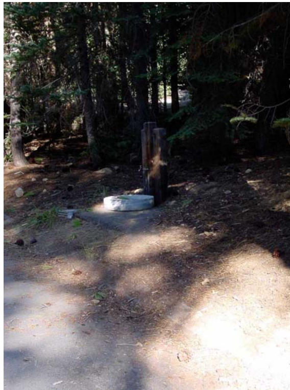
Catavee / Kinnikinnick Campgrounds, Water Spigot - ADA Design, but Inaccessible
