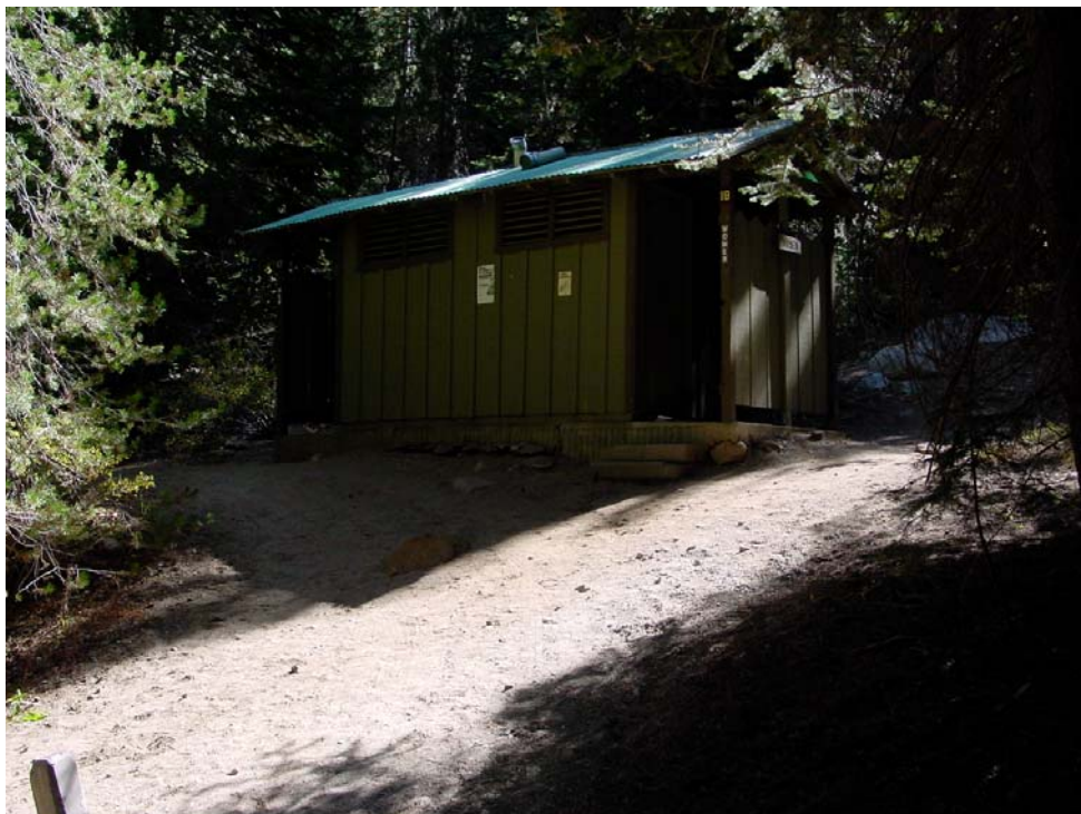
Rancheria Campground, Typical USDA-FS Pit Toilet Facility – Non-ADA Compliant
