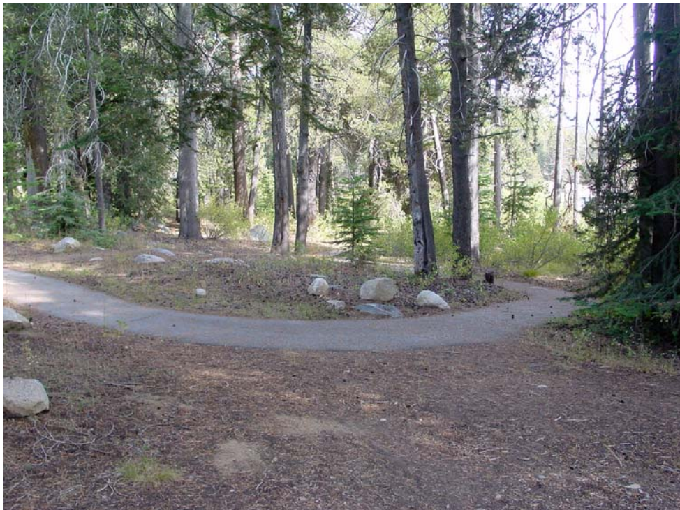
Deer Creek Campground, Paved Pedestrian Path – ADA Compliant
