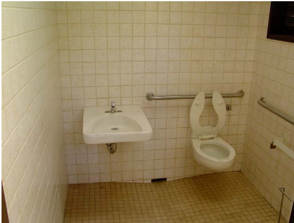
Boat Ramp – Huntington Lake (USDA-FS), Beach Area Restroom Stall – ADA Compliant
