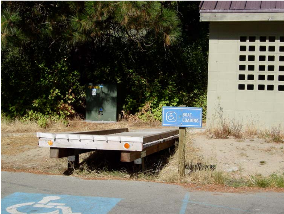
Boat Loading Ramp, Sierra Marina - ADA Compliant
