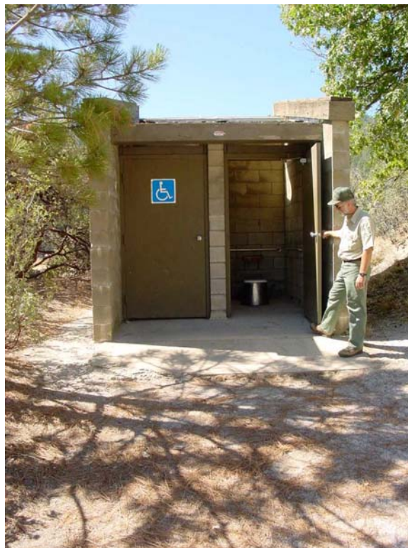
Boat Ramp – Mammoth Pool, Restroom – ADA Identified, but Questionable Accessibility
