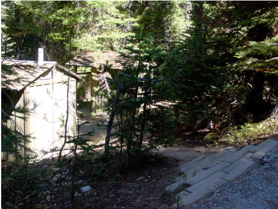
Rancheria Campground, Inaccessible Restrooms
