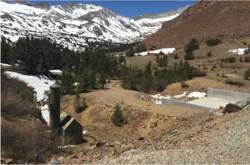
Saddlebag spillway and low-level outlet
