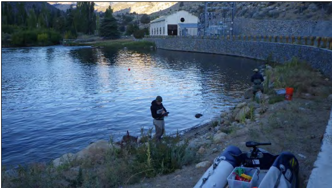
Figure A-37 Forebay 4 overview photo, September 24, 2019
