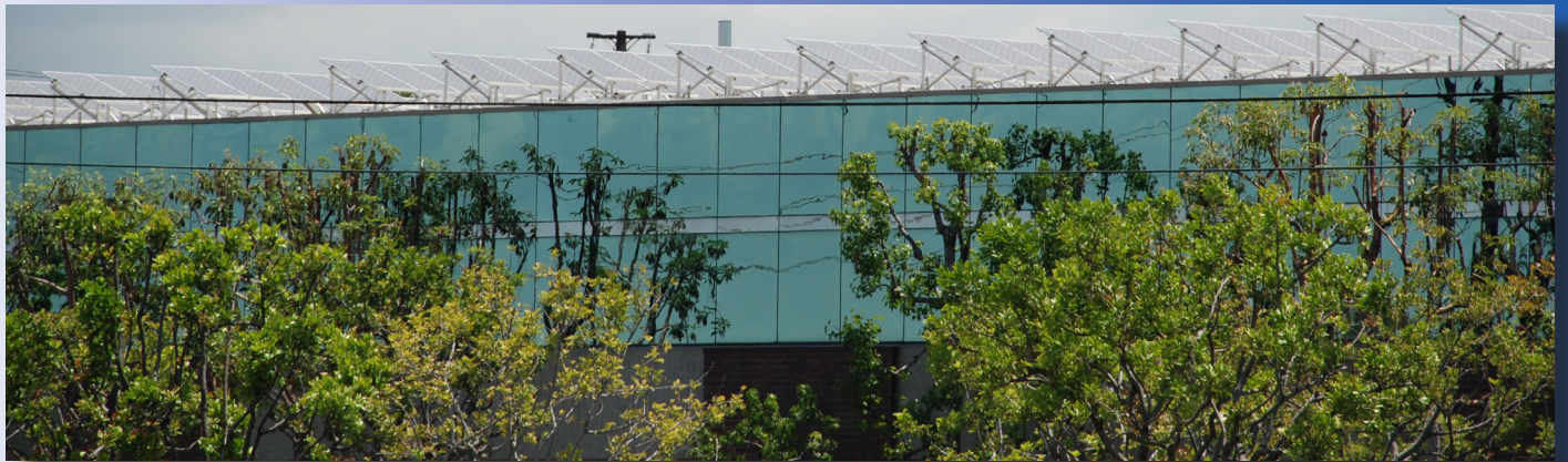
Rooftop solar on an office building
