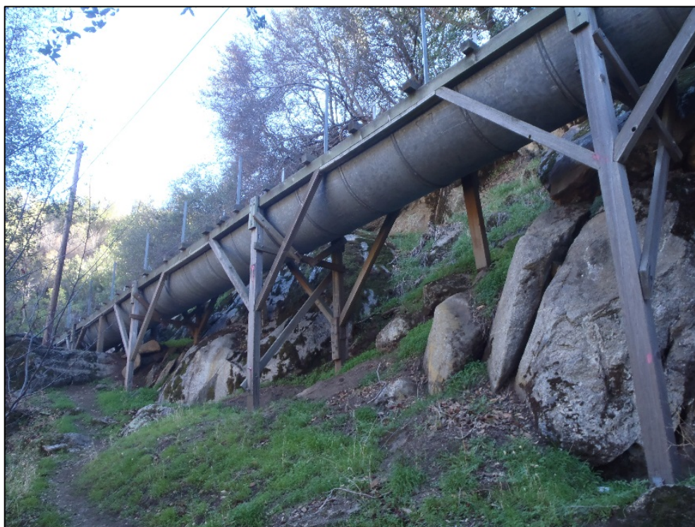
Figure 3.12-1d. Kaweah No. 1 Flowline, typical flume section.
