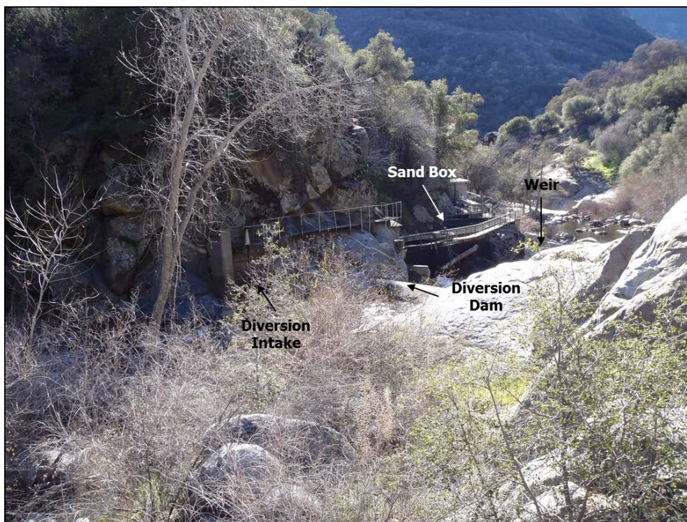
Figure 3.12-1a. Overview of the Kaweah No. 1 Diversion Dam and associated structures on the East Fork Kaweah River.
