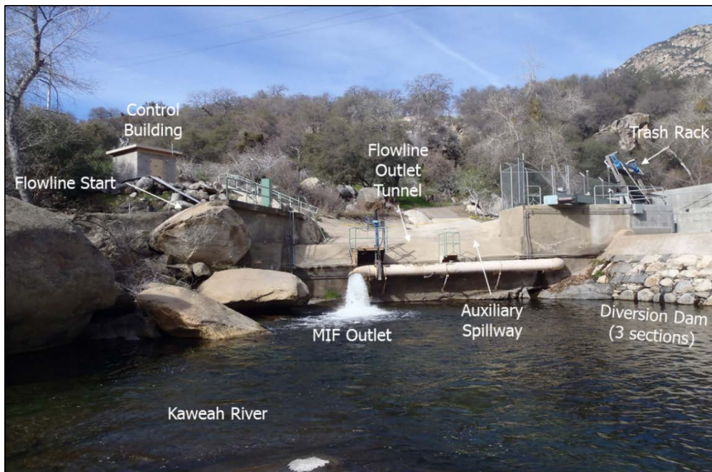
Figure 3.12-1g. Kaweah No. 2 Diversion Dam and associated structures on the Kaweah River.
