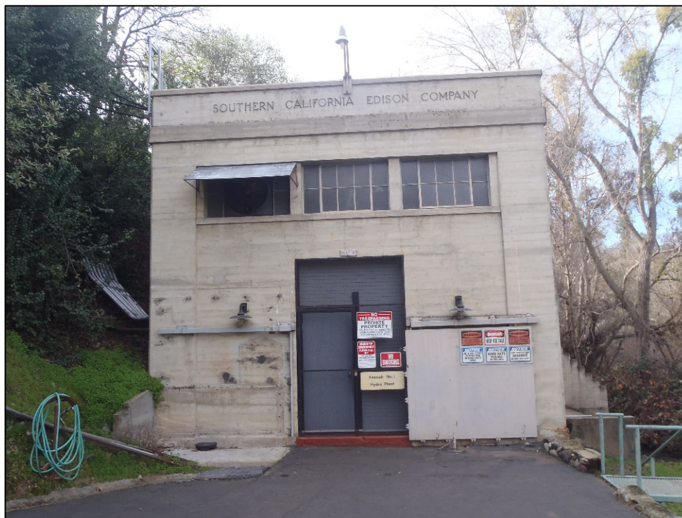
Figure 3.12-1e. Kaweah No. 1 Powerhouse.
