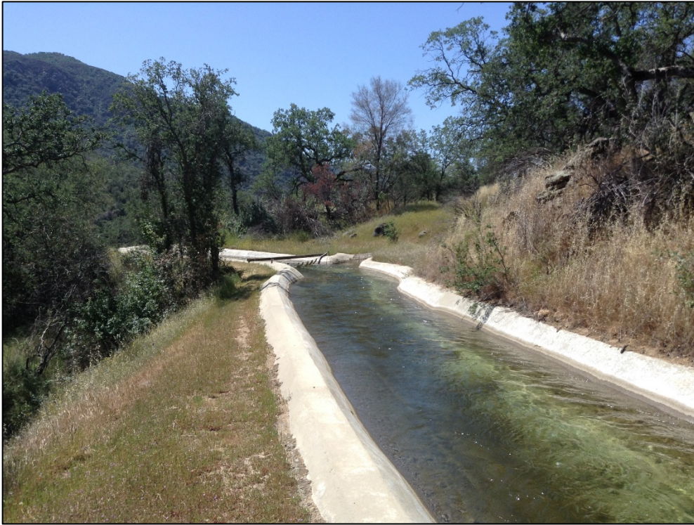
Figure 3.12-1i. Kaweah No. 2 Flowline, typical concrete-lined section.
