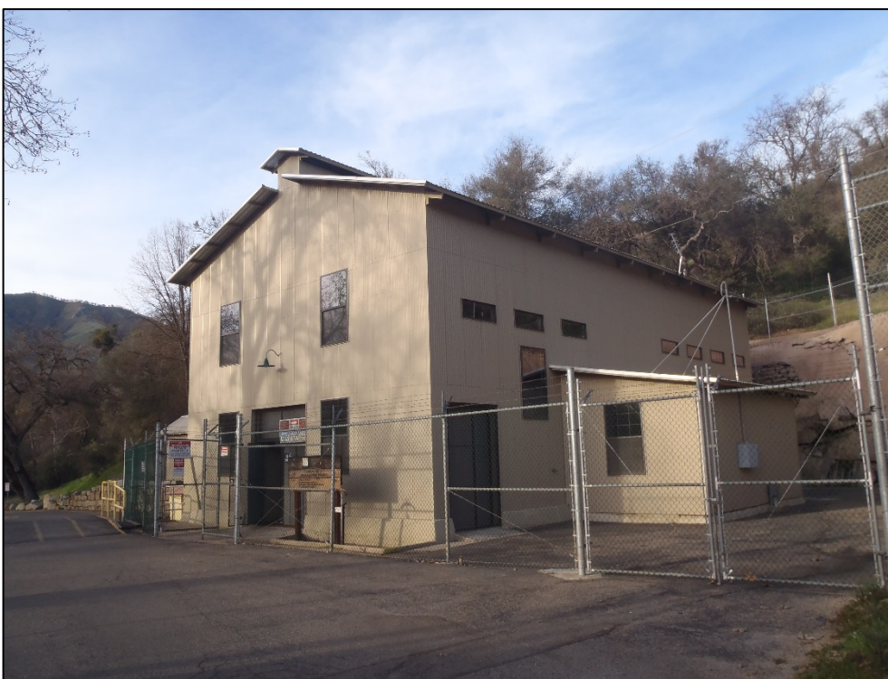
Figure 3.12-1l. Kaweah No. 2 Powerhouse.
