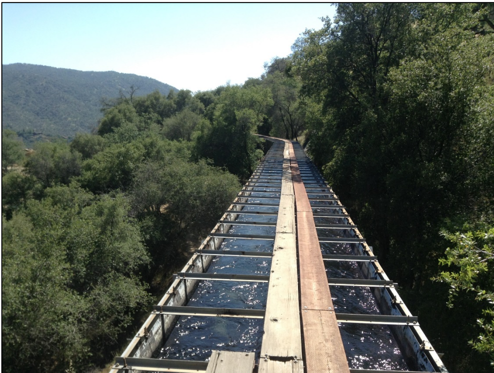
Figure 3.12-1j. Kaweah No. 2 Flowline, typical flume section.
