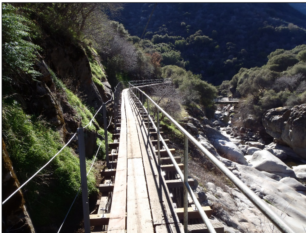
Figure 3.12-1c. Kaweah No. 1 Flowline, typical flume section along East Fork Kaweah River.
