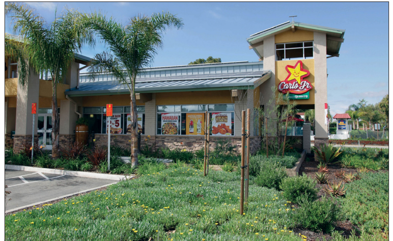
This Carl's Jr. in Carpinteria uses a 12-kW solar energy system that can generate more than 19,200 kWh of electricity annually.
