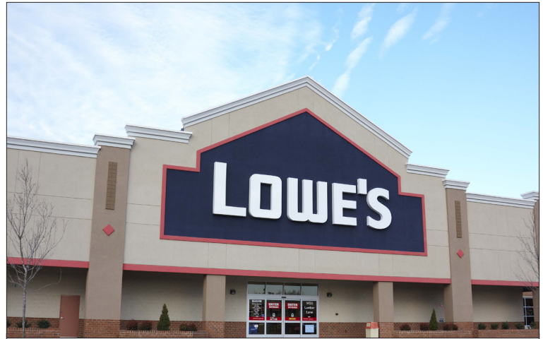
Lowe's recent installation of demand control ventilation systems in about 20 of its stores in SCE's service territory is projected to save nearly 1.5 million kilowatt-hours annually.
