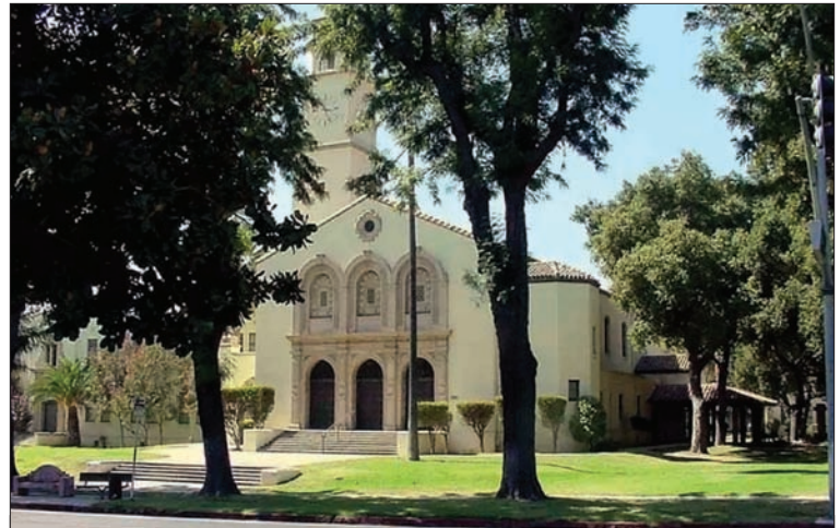
Lighting and computer management software upgrades completed by the Chaffey Joint Union High School District earned the district more than $75,000 in incentives from SCE, with annual energy savings of nearly 919,000 kWh.
