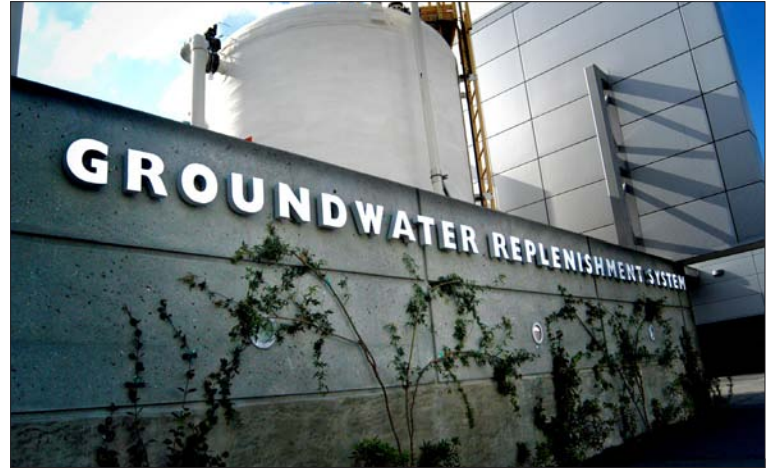
The Orange County Water District worked with SCE to maximize the energy efficiency of its Groundwater Replenishment System facility, earning an incentive of more than $420,000.
