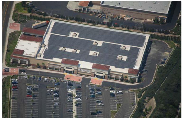
Kohl's operates solar energy systems on more than two dozen stores in SCE's service territory, including this one in Laguna Niguel.
