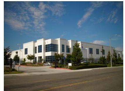
Working with SCE, General Mills upgraded and expanded its Dominguez Hills Customer Service cold storage and shipping facility, with combined savings of more than 1.1 million kWh from the projects.
