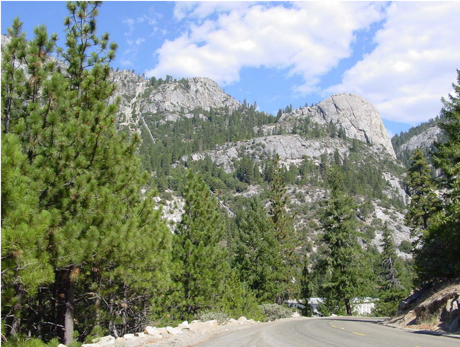
Photo 1. Big Creek No 1 Penstocks (viewed from Huntington Lake Road).
