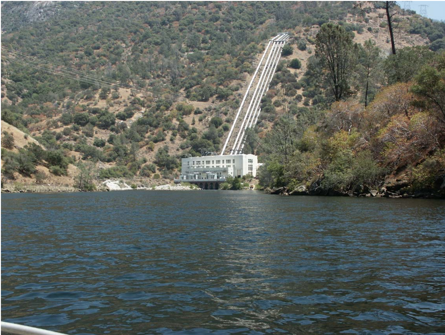
Photo 2. Big Creek No. 3 Powerhouse and Penstocks (viewed from Redinger Lake and Italian Bar Road).
