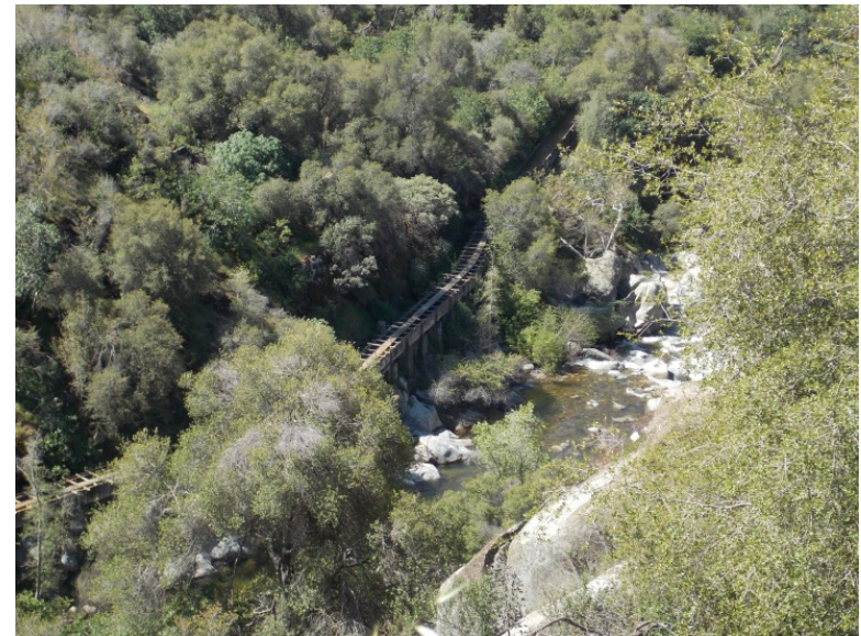
Middle Fork Kaweah River Kaweah No. 3 Flume
