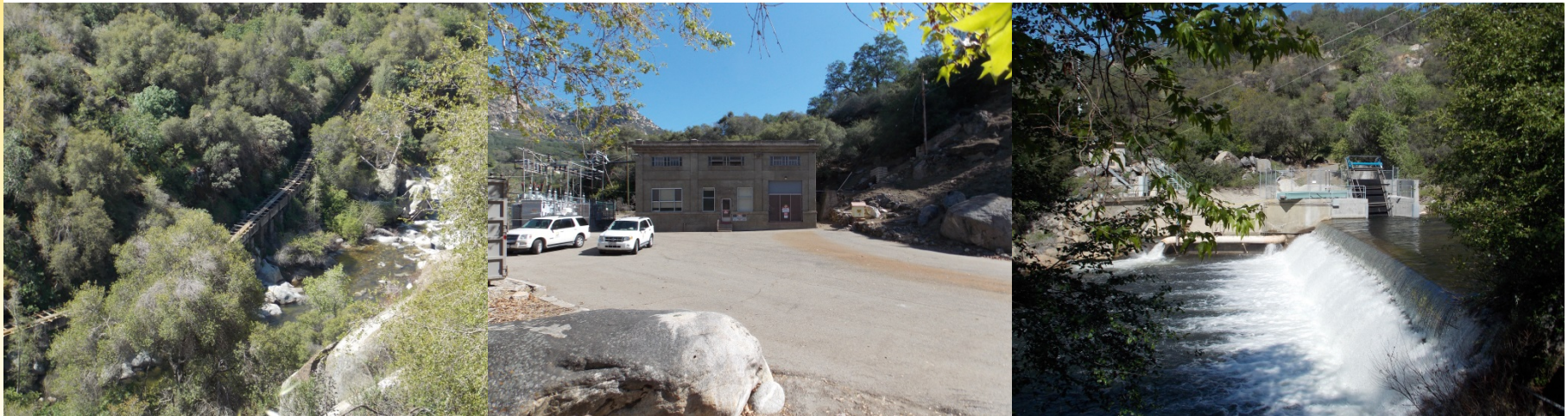
Middle Fork Kaweah River Kaweah No. 3 Flume
