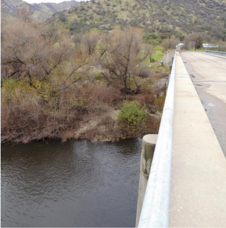
Photo B-32. North Fork Bridge, Downstream Left
