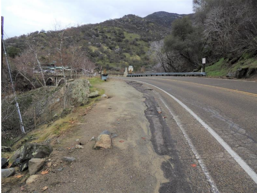
Photo B-11. Gateway Bridge, Roadside Pull-off
