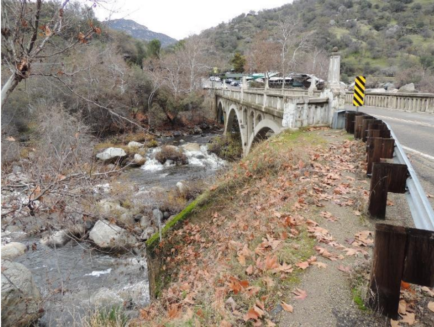
Photo B-9. Gateway Bridge, Downstream Left
