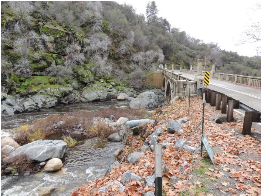
Photo B-8. Gateway Bridge, Upstream Right
