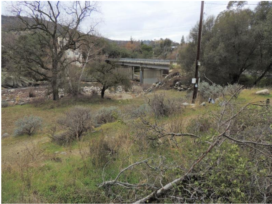
Photo B-21. Dinely Drive, Upstream of Bridge
