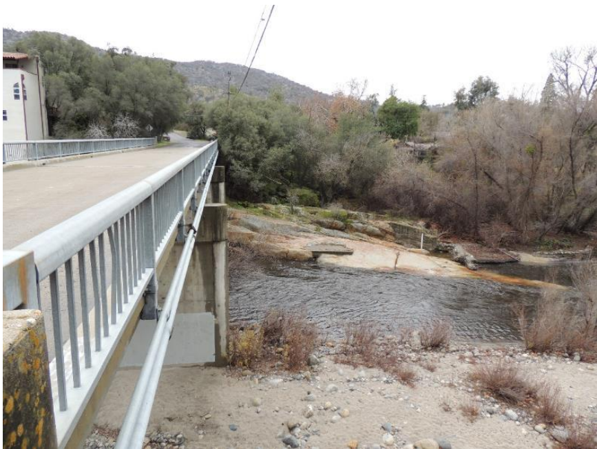
Photo B-20. Dinely Bridge, Downstream Right
