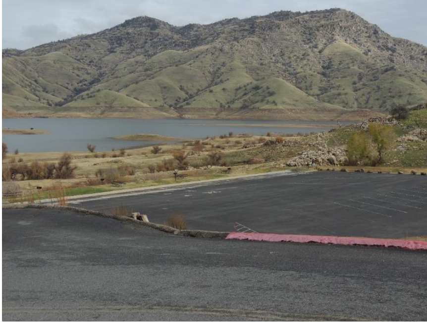
Photo B-39. Lake Kaweah Recreation Area, Parking
