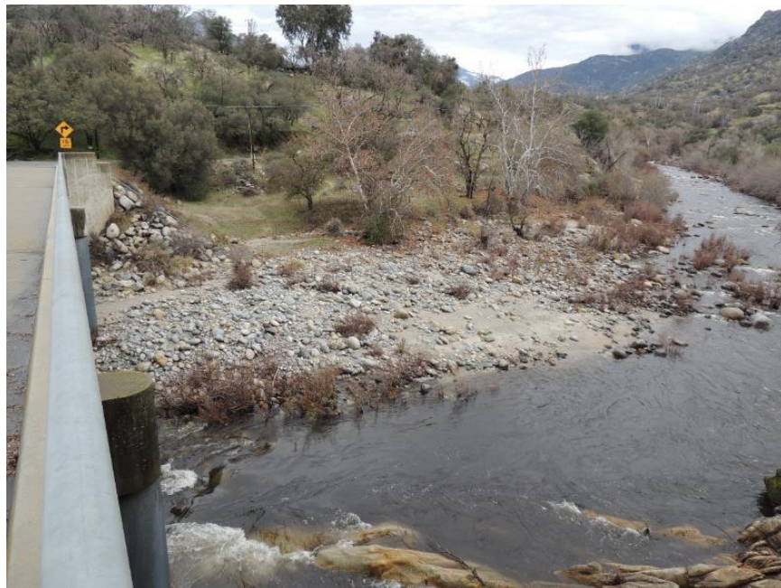
Photo B-17. Dinely Bridge, Upstream Left
