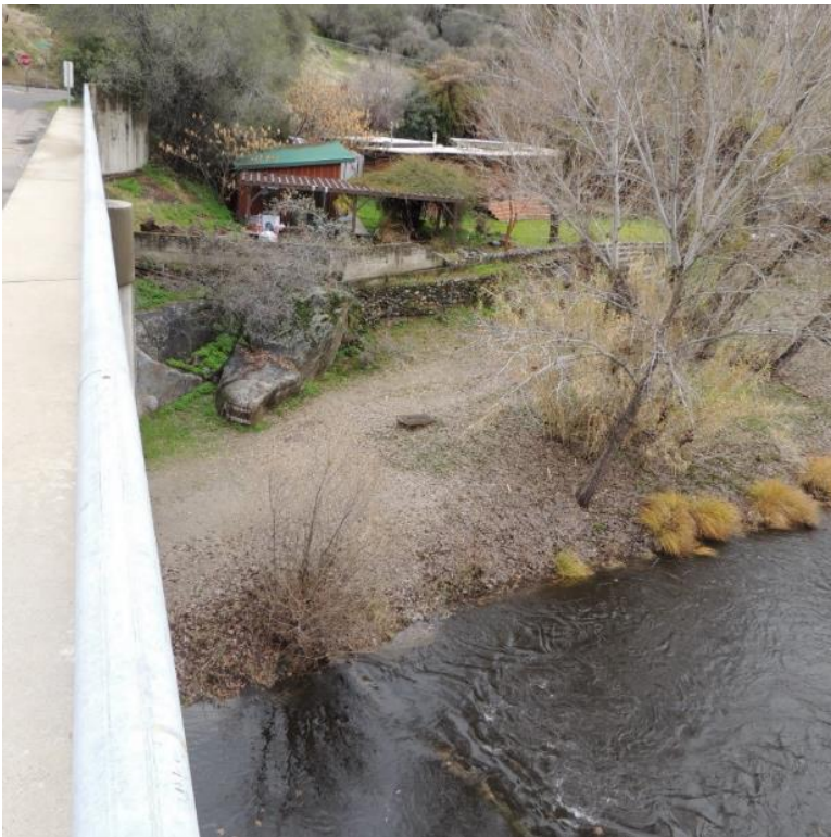
Photo B-33. North Fork Bridge, Downstream Right
