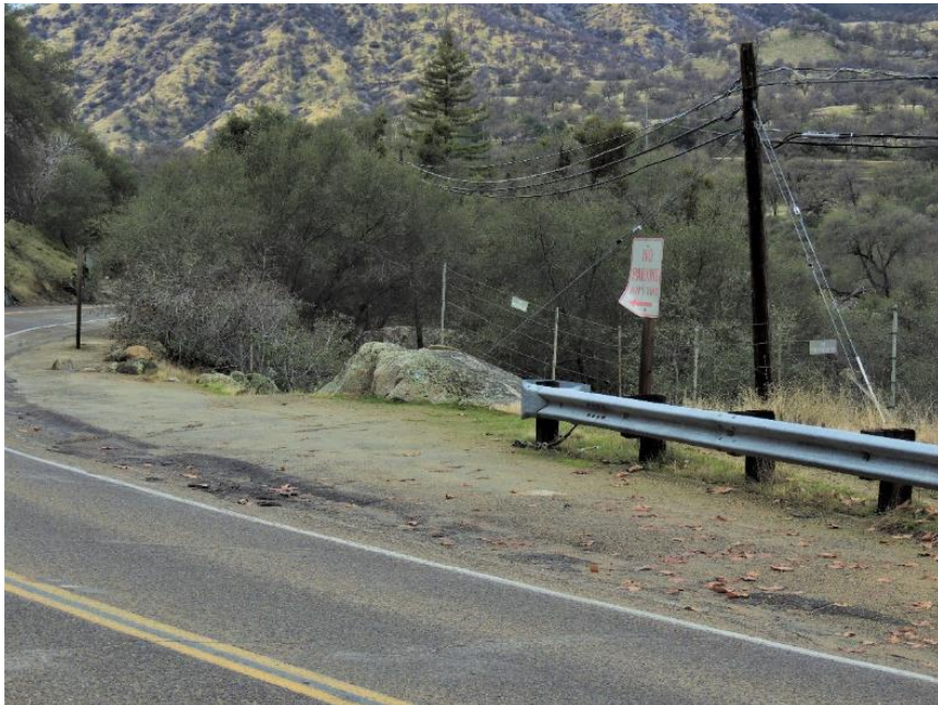
Photo B-12. Gateway Bridge, Roadside Pull-off
