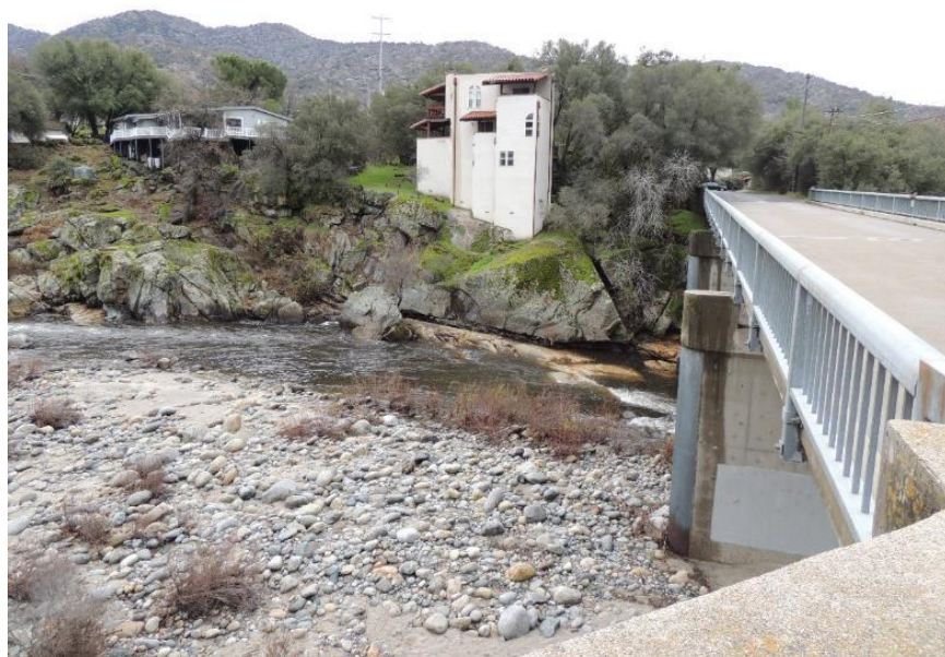
Photo B-18. Dinely Bridge, Upstream Right
