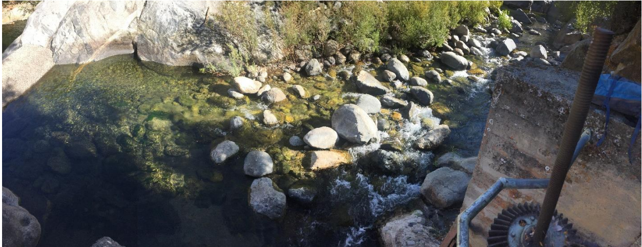
Figure AQ 5-2a. An image of the Kaweah No. 1 Diversion pool sediment deposit, from river left. The diversion dam is visible in the left of the image. Flow is right to left.
