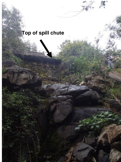
Figure AQ 5-7a. Representative photograph of the upper portion of the drainage chute and natural drainage channel that receives flow from the Kaweah No. 3 Forebay.
