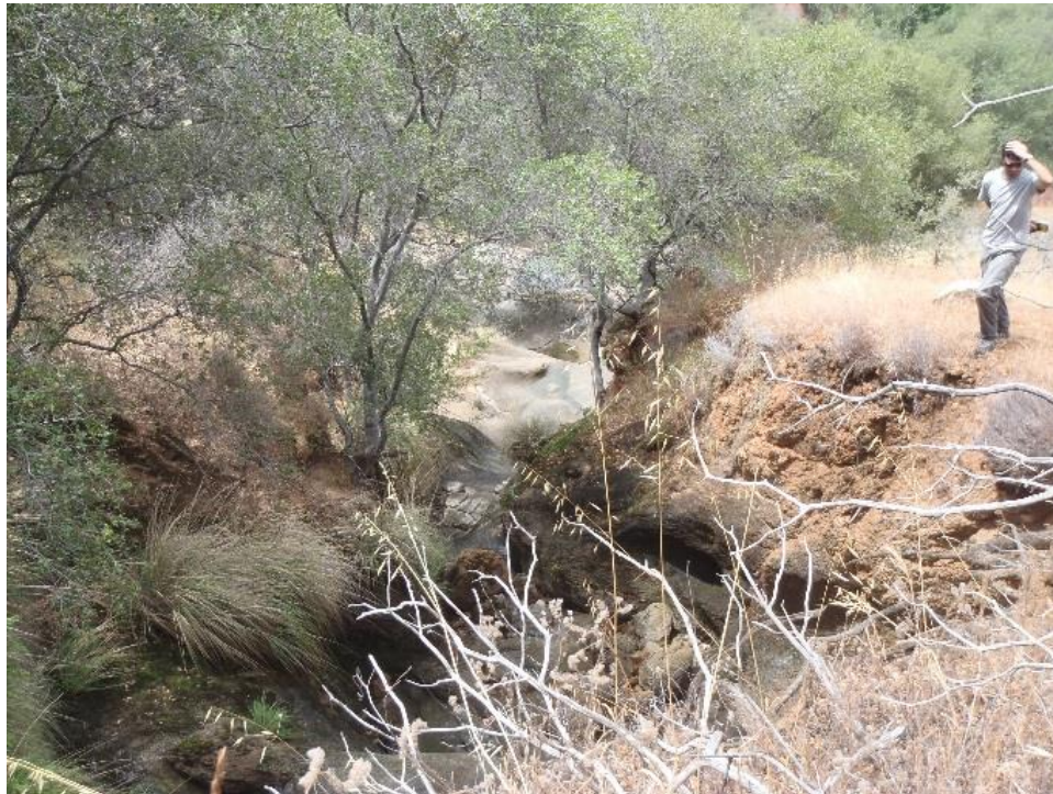
Figure AQ 5-6b. Representative photograph of a down cut section in the natural drainage channel which receives flow from the Kaweah No. 2 Forebay.
