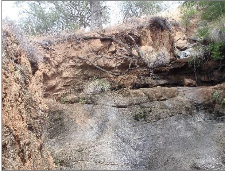
(c) Recent erosion on the side slope of the Kaweah No. 2 natural channel (#1, primary), near the top of the channel.
