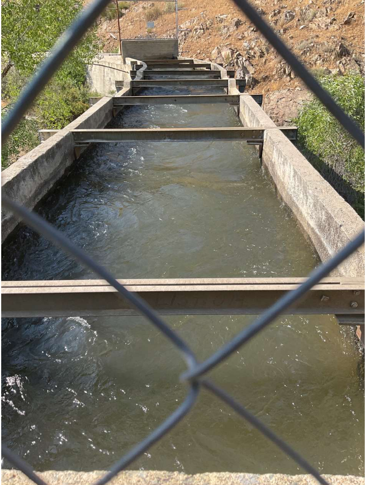
Tunnel at 14 Goldledge .jpg
