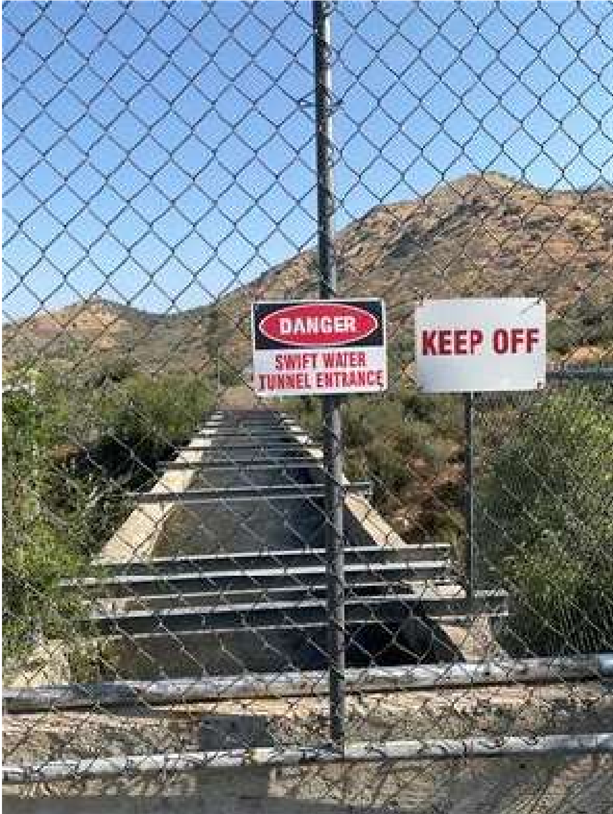
Tunnel at 18 Corral Creek Access (002).jpg
