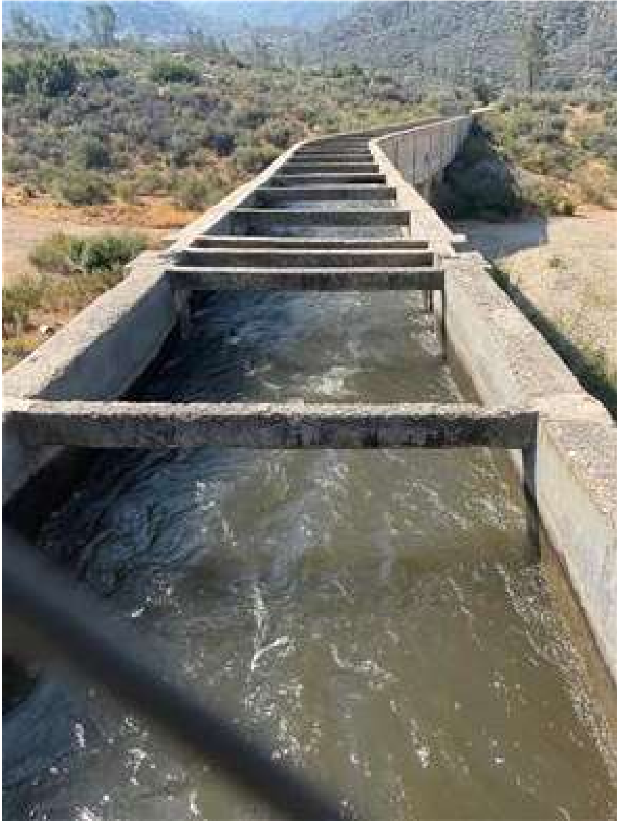
Tunnel at 17Corral Creek North (002).jpg
