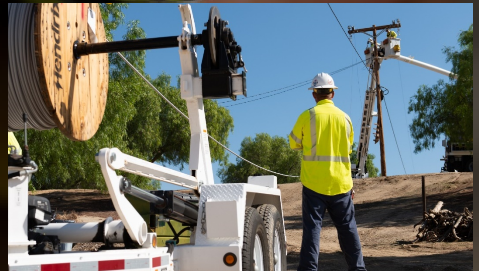
Above photos: SCE crew installing insulated wire
